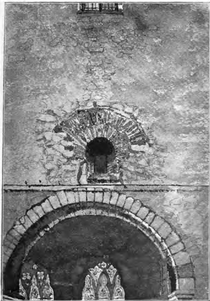
PART OF N. WALL OF NAVE.
