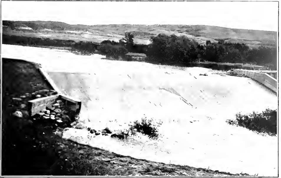
Canadian Pacific Railway Company's Dam in Ross Creek at Irvine.
