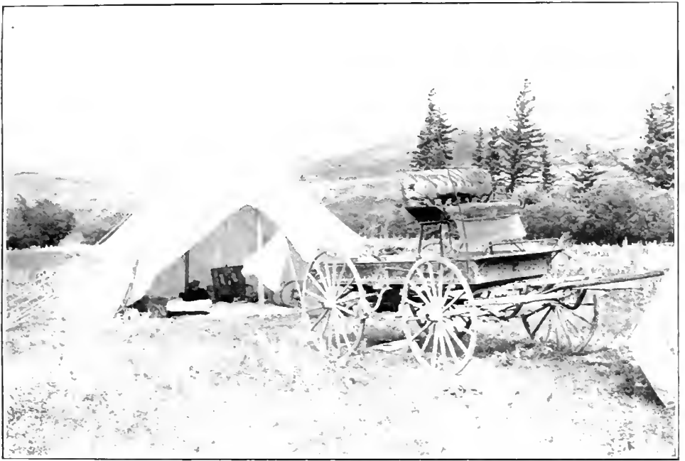
Camp Equipment of the Hydrographer in the Western Cypress Hills district.
