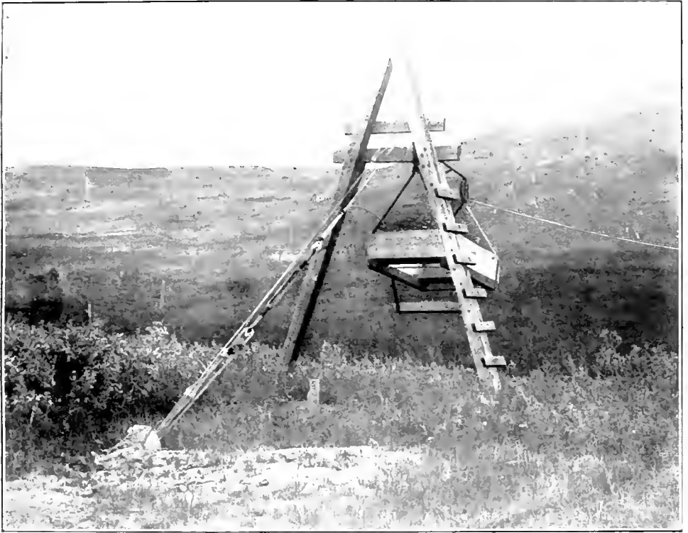
Cable Support and Fastenings at Station on North Branch of Milk River at Peters' Rancho. Taken by F. H. Peters.
