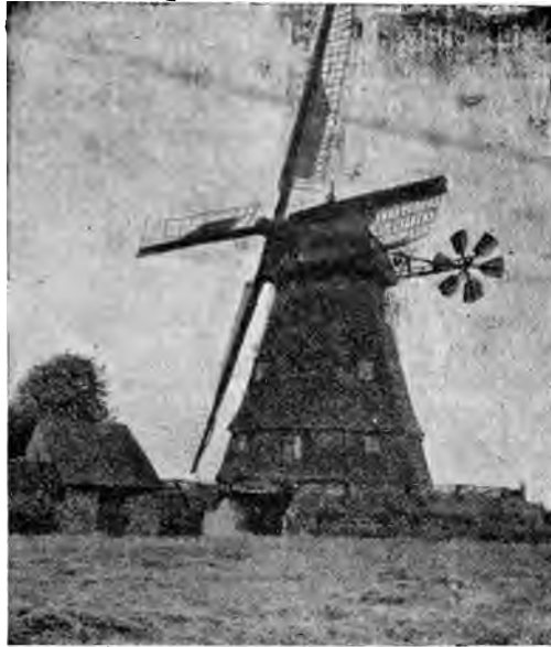
FIG. 3.—Tower Mill with Regulating or Wind Wheel.
