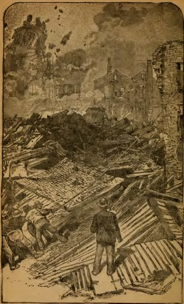
TEARING DOWN HOUSES IN JOHNSTOWN.
